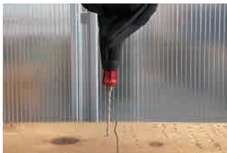
Pilot hole drill
